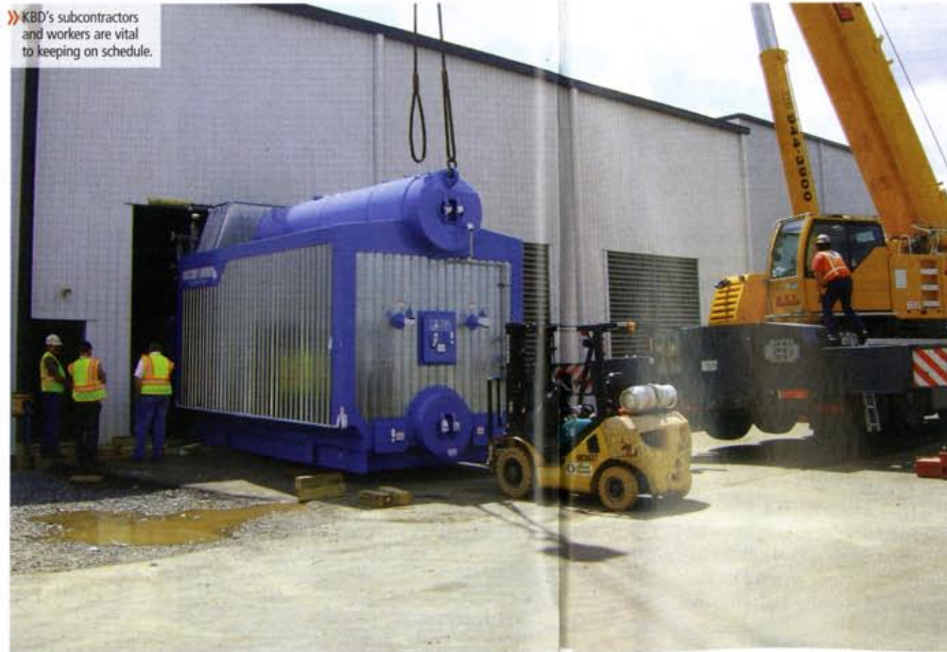
« The project team holds numerous meetings to stay efficient on-site.
